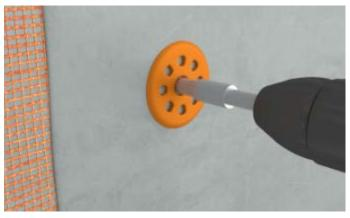
Screw or hammer the fixing into place ensuring the central pin is either flush with the fixing head or slightly recessed. The fixing head should be slightly recessed into the scrim coat face about 1-2mm.
