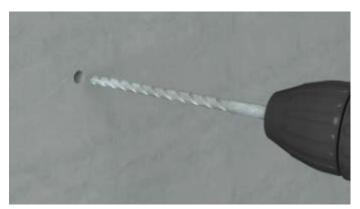
Following the specified fixing pattern, first drill through the basecoat and mesh, insulation and into the masonry substrate with an 8mm diameter drill bit to the appropriate depth.
