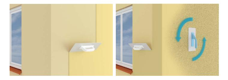
The silicone-acrylic texture coat SOLTHERM AF-P+ 15 or silicone texture coat SOLTHERM SFC-P 15 is applied to the required thicknesses (1.5 mm grain size), using a stainless steel trowel and finished with a plastic float to create a textured finish. The drying time is dependent on weather conditions.
