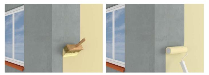
Primer SOLTHERM SNP COLOUR must be applied in with a brush or a paint roller and allowed to completely dry for 4 to 6 hours prior to the application of the silicone topcoat.
