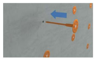
Place the fixing into the pre-drilled hole and push the fixing in until the head of the fixing is flush with the face of the base coat.
