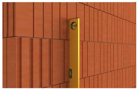
Surface irregularities and cavitiesm (5-15mm) must be made good with SOLTHERM LRC, irregularities ≤5mm can be levelled using SOLTHERM MB or SOLTHERM UB Special
