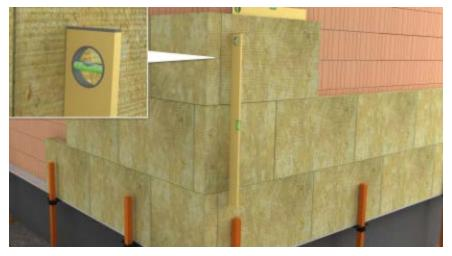
Always ensure that the insulation board are line and level throughout the façade, paying particular attention to external corners.
