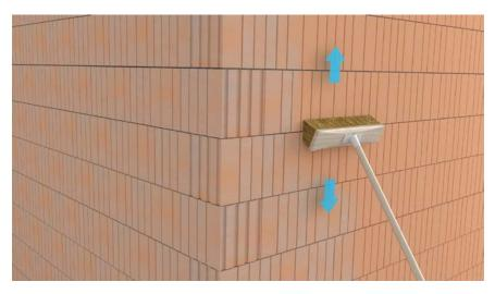
If required, apply FUNGICIDAL WALL WASH to the substrate in accordance with the specification and technical datasheet and allow to dry.
