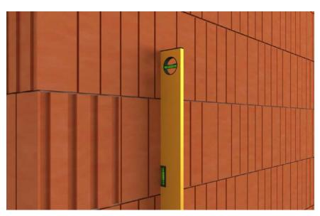
Surface irregularities and cavities (5 - 15 mm) must be made good with SOLTHERM LRC, irregularities  $\leq$  5 mm can be levelled using SOLTHERM MB or SOLTHERM UB Special.
