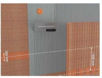
All secondary reinforcing mesh must maintain a minimum overlap of 100 mm with adjacent mesh and all mesh joints must be staggered approximately 500 mm from the joints the first reinforcing mesh application.
