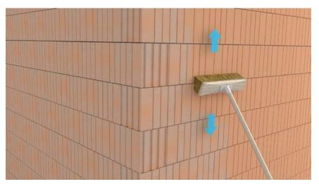
If required, apply FUNGICIDAL WALL WASH to the substrate in accordance with the specification and technical datasheet and allow to dry.
