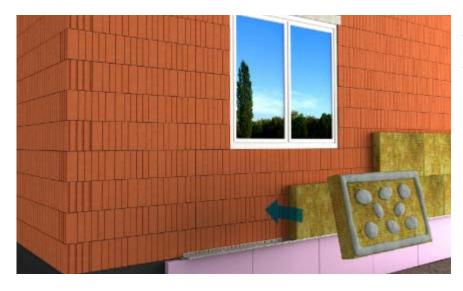
Insulation boards must be placed against the substrate in a brickbond manner achieving a minimum 150 mm stagger with the above/below insulation panel.
