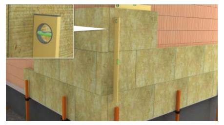
Always ensure that the insulation board are line and level throughout the façade, paying particular attention to external corners.
