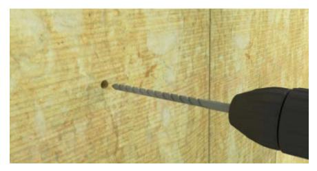
Following the specified fixing pattern, first drill through the insulation and into the masonry substrate with an 8 mm diameter drill bit to the appropriate depth.
