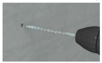
Following the specified fixing pattern, first drill through the basecoat and mesh, insulation and into the masonry substrate with an 8 mm diameter drill bit to the appropriate depth.
