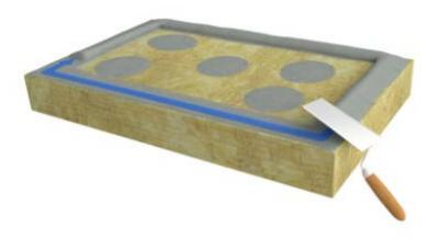
Once the contact layer is applied, apply further insulation adhesive to the perimeter and where the dabs are located.
