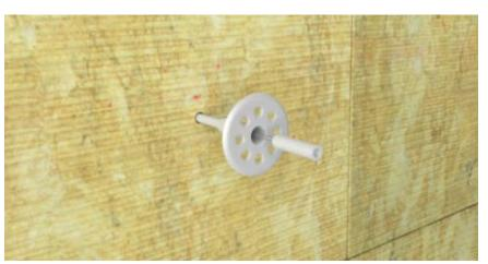
Screw or hammer (depending on fixing specification) the fixing into place ensuring the central pin is either flush with the fixing head or slightly recessed. The fixing head should be slightly recessed into the insulation face about 1-2 mm.
