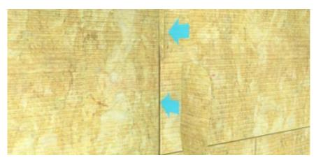
Any gaps between adjacent insulation panels must be filled with mineral wool slithers.
