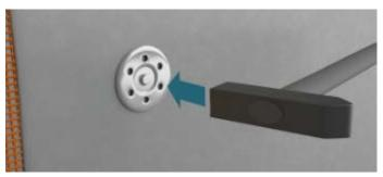
Using a hammer, gently hit the fixing centrally until it is recessed within the mesh and base coat approx. 1-2 mm. While the base coat is still wet for ULTIMATE A1 DASH, place a mesh patch (100x100mm) over the fixing head and smooth over with additional base coat if required.
