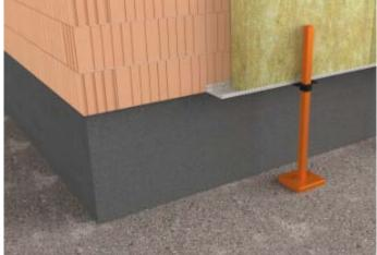
Due to the weight of the mineral wool insulation, it may be a requirement to temporarily support the SOLTHERM STARTER TRACK.
