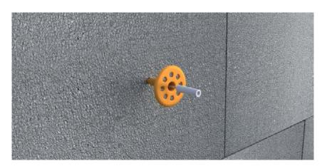
Screw or hammer (depending on fixing specification) the fixing into place ensuring the central pin is either flush with the fixing head or slightly recessed. The fixing head should be slightly recessed into the insulation face about 1 - 2 mm.
