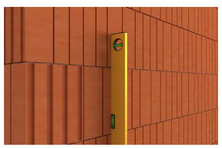
Surface irregularities and cavities (5-15mm) must be made good with SOLTHERM LRC, irregularities ≤5mm can be levelled using SOLTHERM UB or SOLTHERM UB Special.
