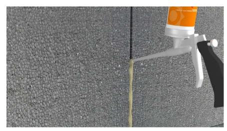
Any gaps between adjacent insulation panels must be filled with SOLTHERM PM-L FOAM or EPS off-cuts.
