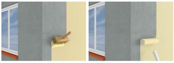
Primer SOLTHERM SNP COLOUR is applied in with a brush or a paint roller and allowed to completely dry for 4 to 6 hours prior to the application of the topcoat.
