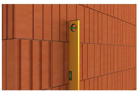
Surface irregularities and cavities (5-15mm) must be made good with SOLTHERM LRC, irregularities  $\leq$  5 mm can be levelled using SOLTHERM UB or SOLTHERM UB Special.
