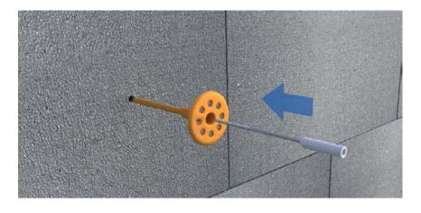
Place the fixing into the pre-drilled hole and push the fixing in until the head of the fixing is flush with the face of the insulation.
