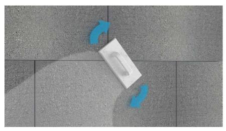
if required, the surface of the EPS can be rasped to ensure the EPS line & level, prior to proceeding with the installation of the system.
