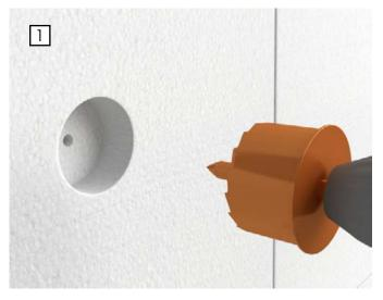
Following the specified fixing pattern, firstdrill through the insulation and into themasonry substrate with an 8 mm or 10 mm diameter drill bit (subject to a fixing) to the appropriate depth.
