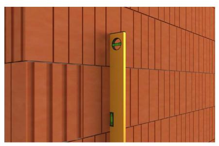
Surface irregularities and cavities (5 - 15 mm) must be made good with SOLTHERM LRC, irregularities  $\leq$  5 mm can be levelled using SOLTHERM UB or SOLTHERM BC-P Quick.
