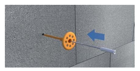
Place the fixing into the pre-drilled hole and push the fixing in until the head of the fixing is flush with the face of the insulation.
