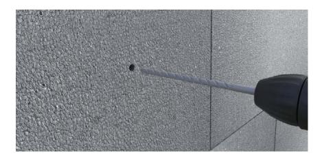
Following the specified fixing pattern, first drill through the insulation and into the masonry substrate with an 8 mm or 10 mm diameter drill bit (subject to a fixing) to the appropriate depth.
