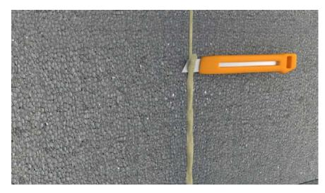
Once fully cured, excess SOLTHERM PM-L FOAM must be removed with a knife to ensure it is flush with the surface of EPS boards.
