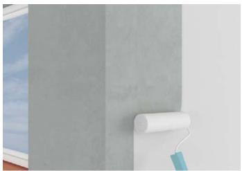
Primer SOLTHERM SNP COLOUR is applied in (if specified) with a brush or a paint roller and allowed to completely dry for 4 to 6 hours prior to the application of the topcoat.
