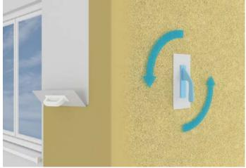
The silicone-acrylic texture coat SOLTHERM AF-P+ 15 or silicone texture coat SOLTHERM SFC-P 15 is applied to the required thicknesses (1.5 mm grain size), using a stainless steel trowel and finished with a plastic float to create a textured finish. The drying time is dependent on weather conditions.
