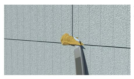
Once fully cured, excess SOLTHERM PM-L FOAM must be removed with a knife to ensure it is flush with the surface of ICF EPS boards.
