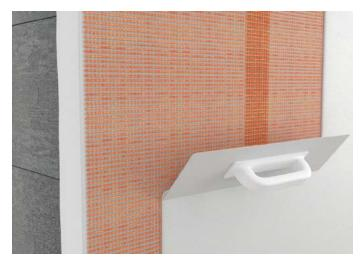
Allow the basecoat to dry for approximately 24 hours before applying a tight slurry coat 1-2 mm. The overall thickness of the basecoat should be between 3-5 mm.
