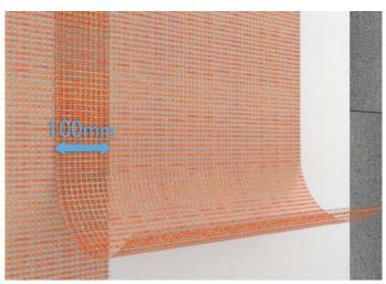
While the base coat is thoroughly wet, using an 8-10 mm notch trowel, apply a vertical notch. Gently lay the reinforcement mesh into the wet base coat, keeping the mesh in the top third of the material and ensuing the mesh has a minimum lap of 100 mm with all adjacent meshes.
