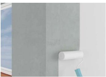
Primer SOLTHERM SNP COLOUR is applied in (if specified) with a brush or a paint roller and allowed to completely dry for 4 to 6 hours prior to the application of the topcoat.
