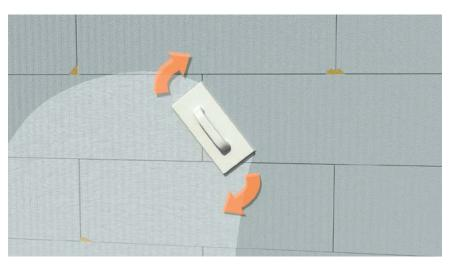
Where approved by the ICF system manufacturer, it is recommended that the outer surfaces of the EPS insulation panels, are lightly rasped with coarse sandpaper or an abrasive float rasp for EPS, to remove dust from the EPS surfaces.
