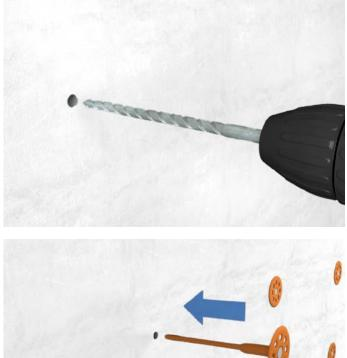
Following the specified fixing pattern, first drill through the basecoat and mesh, insulation and into the masonry substrate with an 8mm diameter drill bit to the appropriate depth.
