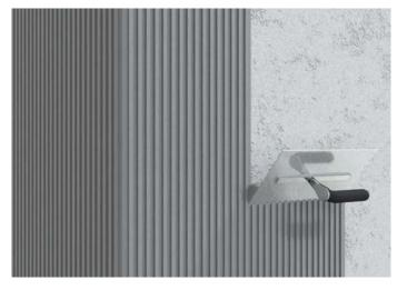
Apply SOLTHERM SE to the cured base coat with an 8mm notched trowel, notching in various directions to allow optimal adhesion strength.
