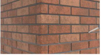
Place SOLTHERM KL pointing mortar into a suitable pointing gun. Using the pointing gun, fill the brick joints with SOLTHERM KL, fully filling the joint.
