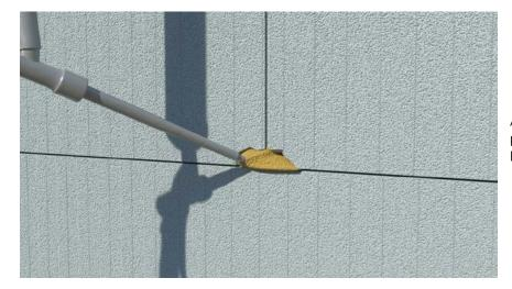
Any gaps between adjacent ICF insulation panels must be filled with SOLTHERM PM-L FOAM or EPS off-cuts.
