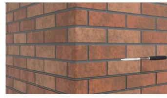
Once SOLTHERM KL pointing mortar has sufficiently picked up but remains ,green', point the mortar to the required method. Once complete, the walls are to brushed down with a soft brush at an approximate 45° angle, removing excess pointing mortar and cleaning the face of the brick slips.
