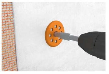
Screw or hammer the fixing into place ensuring the central pin is either flush with the fixing head or slightly recessed. The fixing head should be slightly recessed into the scrim coat face about 1-2mm.
