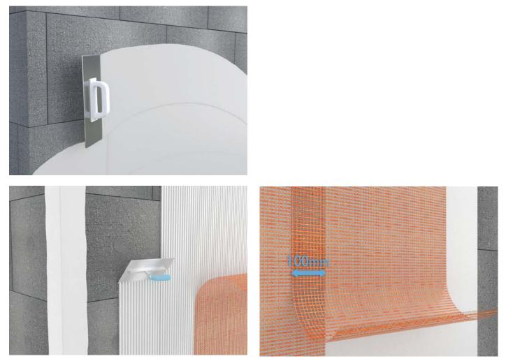
While the base coat is thoroughly wet, using an 8-10 mm notch trowel, apply a vertical notch. Gently lay the reinforcement mesh into the wet base coat, keeping the mesh in the top third of the material and ensuing the mesh has a minimum lap of 100 mm with all adjacent meshes.
