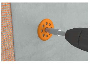
Screw or hammer the fixing into place ensuring the central pin is either flush with the fixing head or slightly recessed. The fixing head should be slightly recessed into the scrim coat face about 1-2mm.
