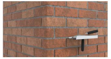
Using a handboard/hawk, offer SOLTHERM KL pointing mortar up the joint and using an appropriate trowel, fill the brick joints with SOLTHERM KL, fully filling the joint.
