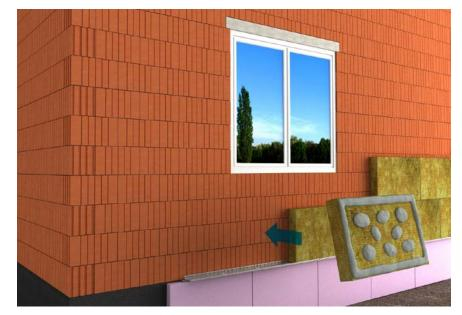
Insulation boards must be placed against the substrate in a brickbond manner achieving a minimum 150mm stagger with the above/below insulation panel.
