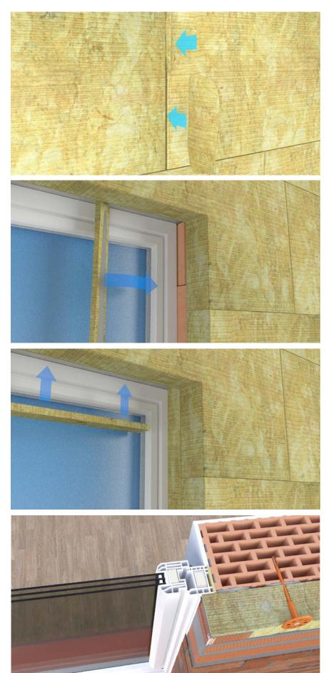
Any gaps between adjacent insulation panels must be filled with mineral wool slithers.
