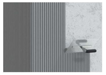
Apply SOLTHERM E or SOLTHERM SE to the cured base coat with an 8mm notched trowel, notching in various directions to allow optimal adhesion strength.
