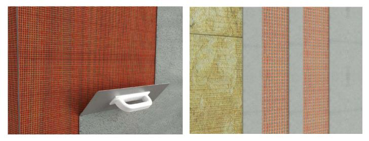
Allow the base coat to dry for approximately 24 hours before applying a tight slurry coat 1-2mm if required. The overall thickness of the base coat for DECO P BRIQ system should be between 4-6mm with two reinforcing meshes.
