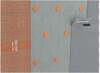
Apply a further coat of SOLTHERM MB or SOLTHERM UB Special at 1-2mm thick and lay through Standard SOLTHERM MESH ensuring no mesh is visible and is fully encapsulated in the base coat.
