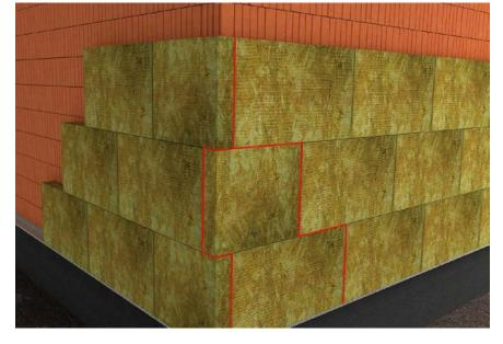
External corners are formed as per a brickwork corner, ensuring a full brickbond.
