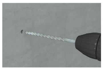
Following the specified fixing pattern, first drill through the basecoat and mesh, insulation and into the masonry substrate with an 8mm diameter drill bit to the appropriate depth.
