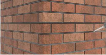
Place SOLTHERM KL pointing mortar into a suitable pointing gun. Using the pointing gun, fill the brick joints with SOLTHERM KL, fully filling the joint.
