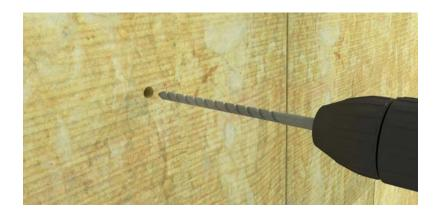
Following the specified fixing pattern (minimum of 1 or 2 per insulation board), first drill through the insulation and into the masonry substrate with an 8mm diameter drill bit to the appropriate depth.
