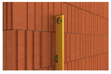
Surface irregularities and cavities (5-15mm) must be made good with SOLTHERM LRC, irregularities <5mm can be levelled using SOLTHERM MB or SOLTHERM UB Special.
