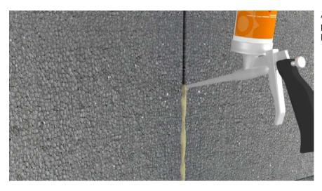
Any gaps between adjacent insulation panels must be filled with SOLTHERM PM-L FOAM or EPS off-cuts.
